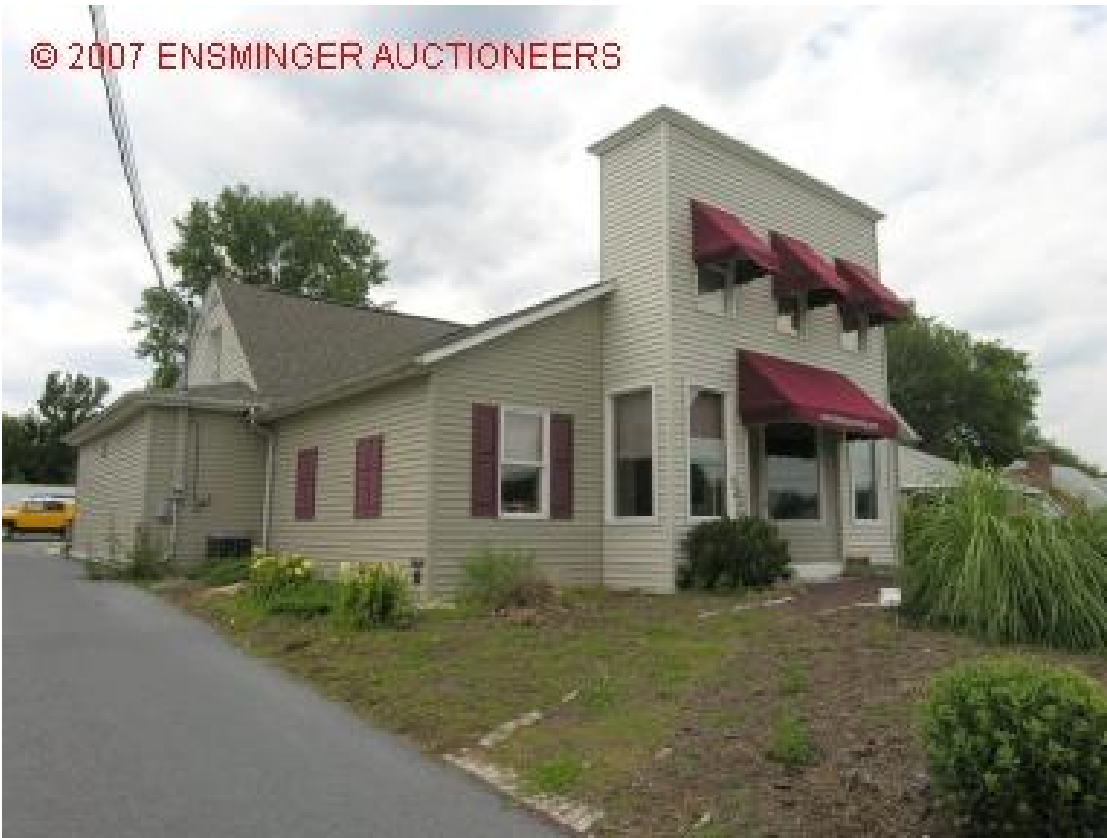
Front of building and left side. Exit driveway.
