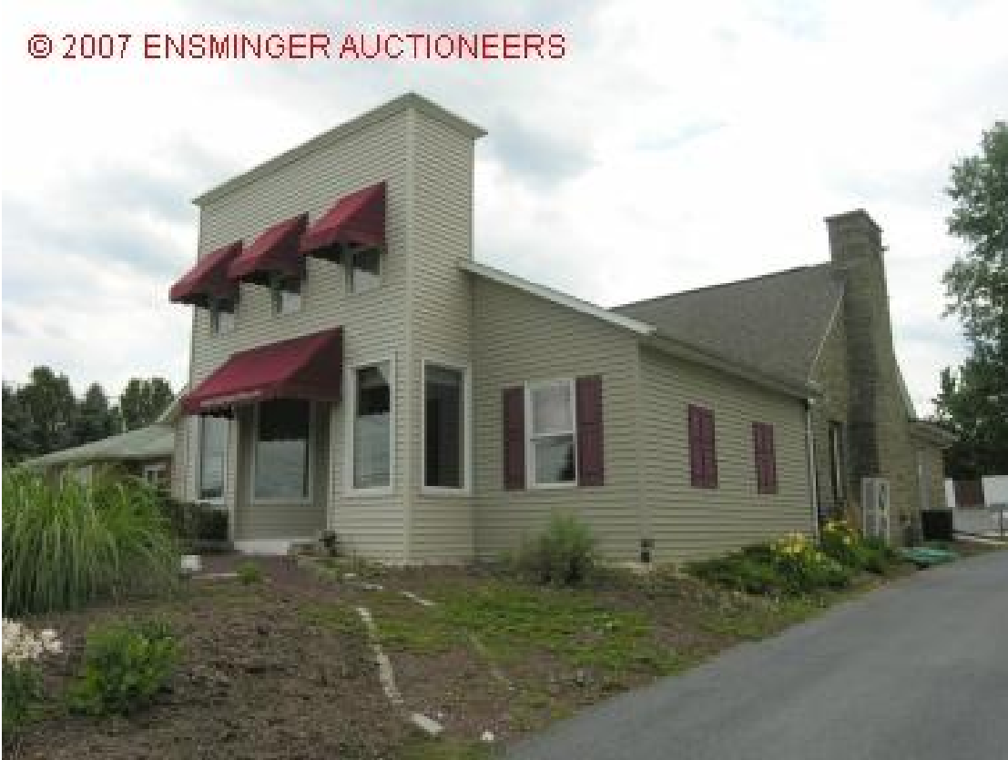
Front of building and right side. Entrance driveway.
