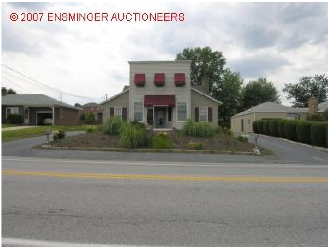
Front of the building. Entrance driveway is on the right, exit driveway is on the left.
